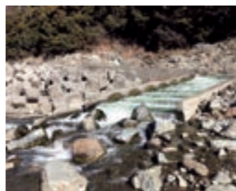
Fishway in TOSHIMA Weir
